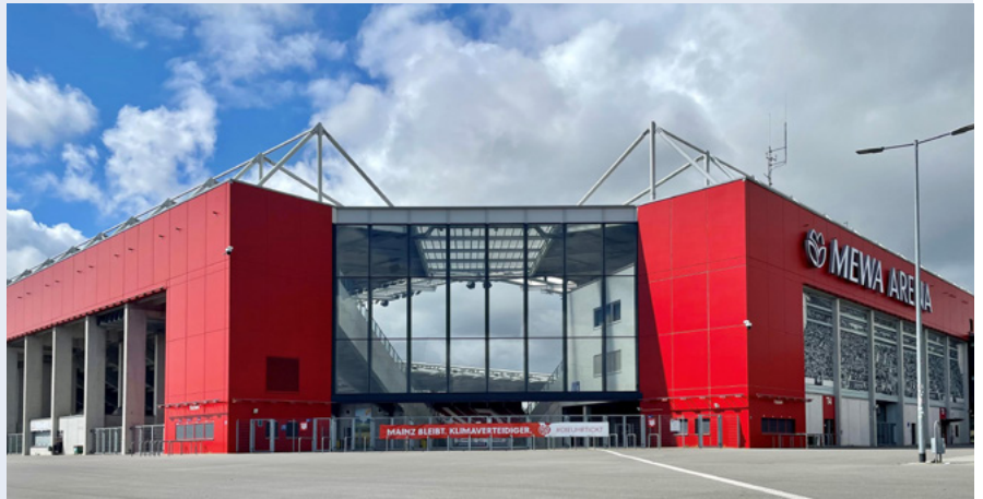
The IT department must be in top form in order for everything to run smoothly in a football league stadium.
