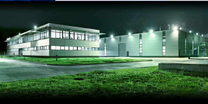
JOYSONQUIN's networks are protected against illegal access around the clock
